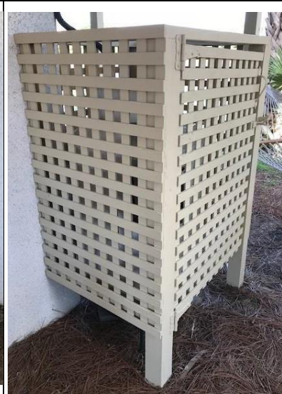
Figure 7c Propane Tank Enclosure (left side and access door)
