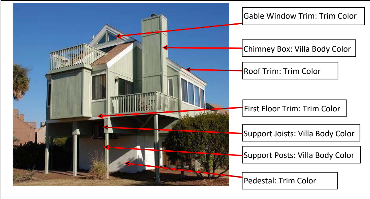
Figure B-1 Master Bedroom / Deck Side of Villa
