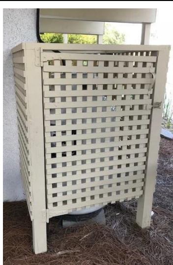
Figure 7a Propane Tank Enclosure Access Door
