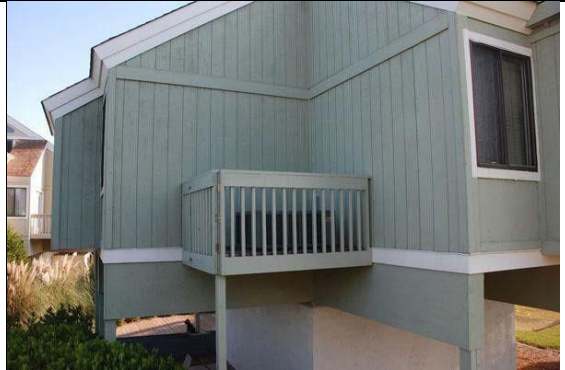
Figure 7b-2 HVAC Stand
