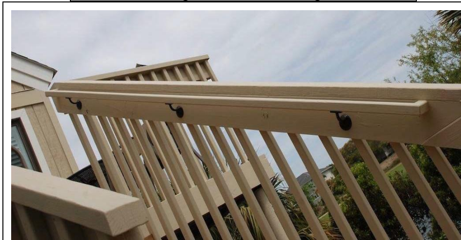
Figure 4c-4 Railing, Balusters, and Stringers
