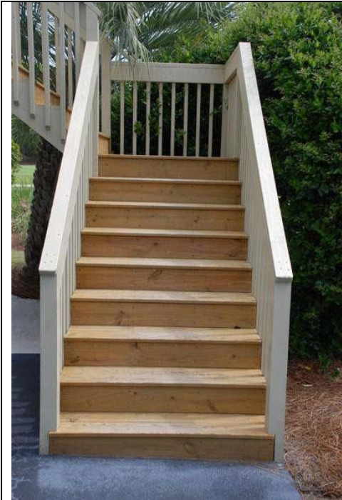
Figure 4c-1 Stairway with Full Risers
