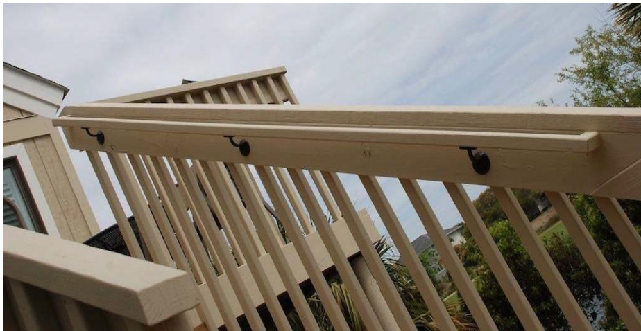
Figure 4c-4 Railing, Balusters, and Stringers
