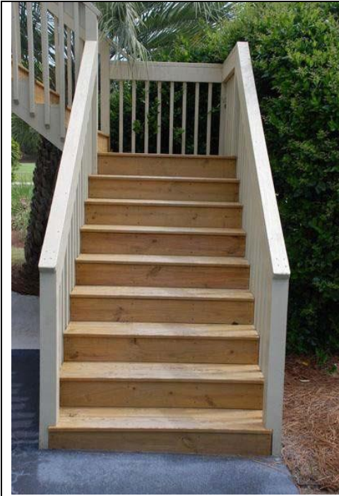
Figure 4c-1 Stairway with Full Risers
