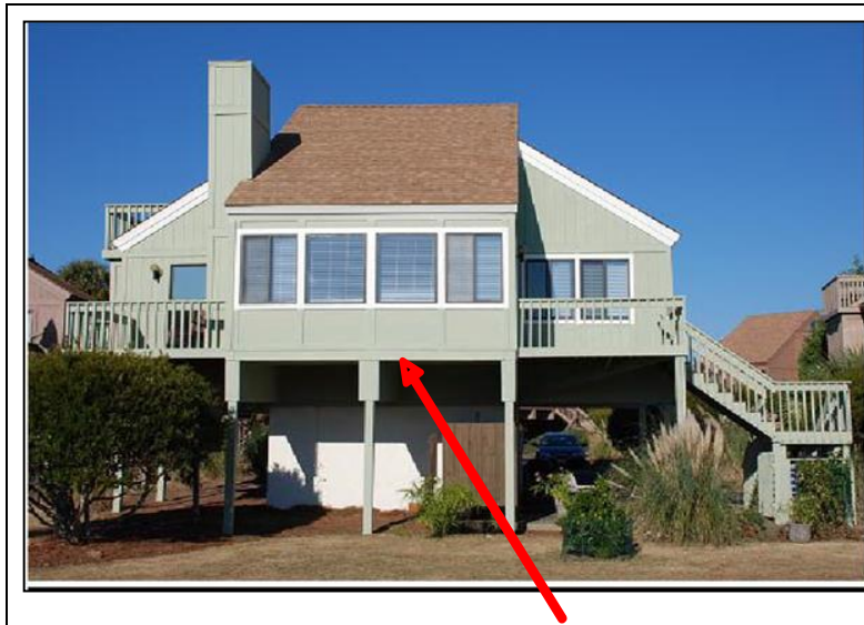
Figure B-7 Depiction of Living Room Wall First Floor Trim
