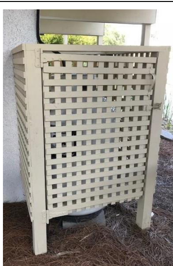
Figure 7a Propane Tank Enclosure Access Door
