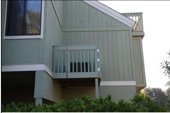
Figure 7b-1 HVAC Stand
