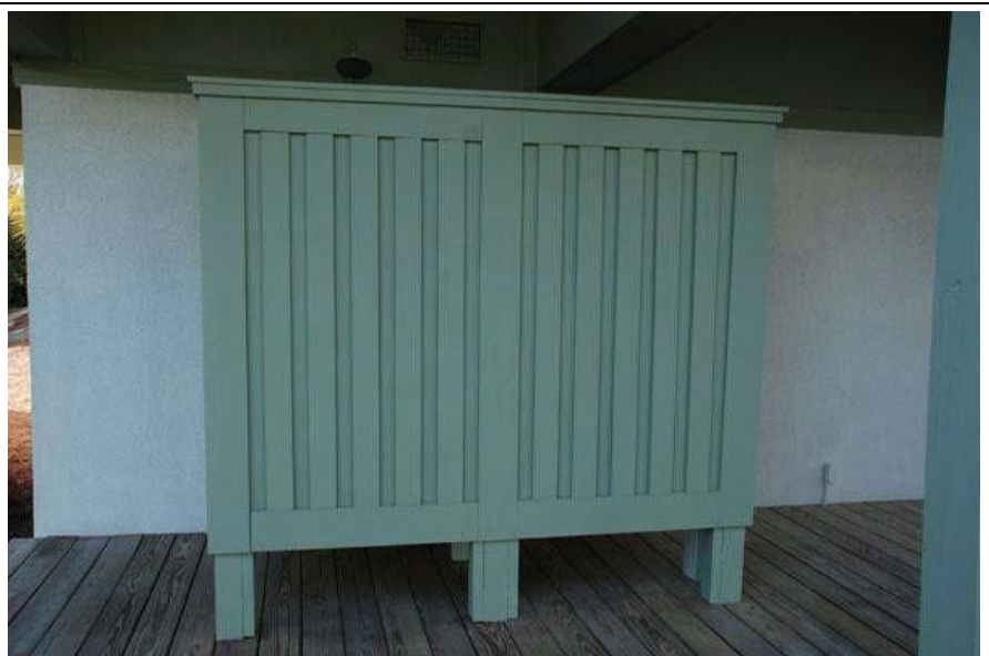
Figure 7e Exterior Shower Enclosure
