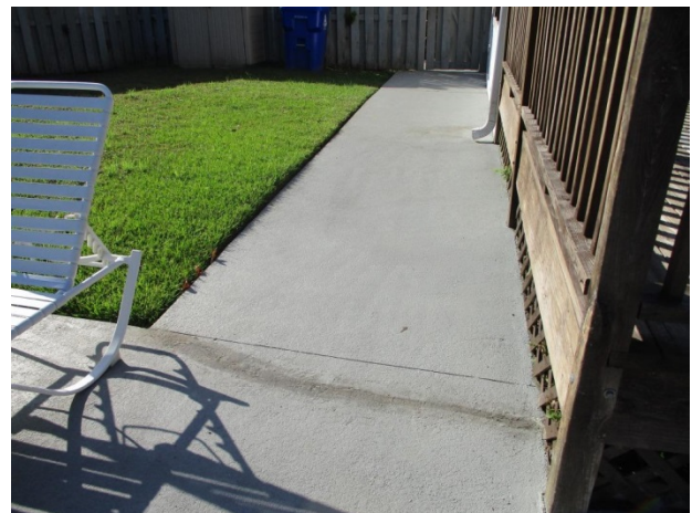
Pool deck overview
