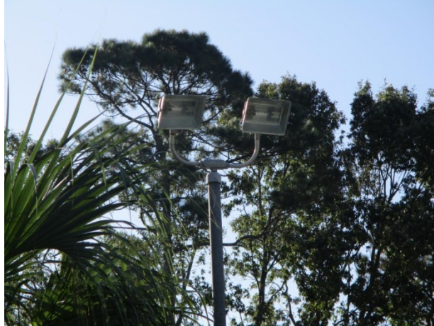
Typical light pole and fixture
