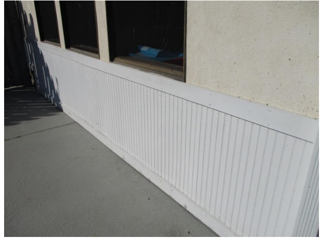
Clubhouse exterior wood siding overview
