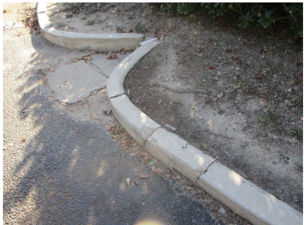
Concrete curb overview
