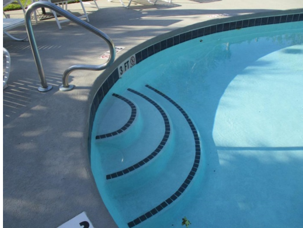
Plaster finish and tile at pool entrance stairs
