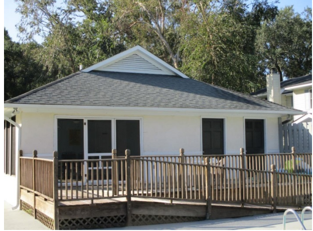
Clubhouse roof overview
