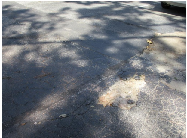
Pavement deterioration
