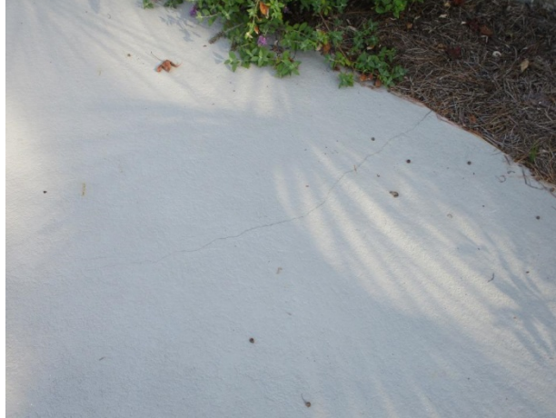
Minor crack in deck
