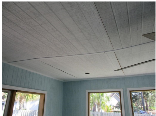
Deflected wood ceiling of sun room
