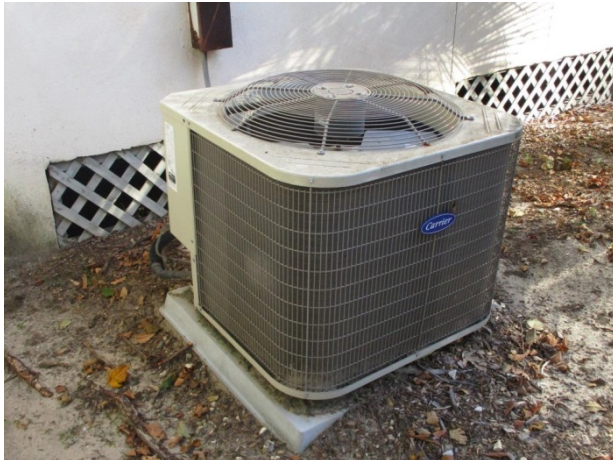
Clubhouse condensing unit
