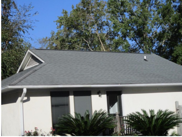
Clubhouse roof overview
