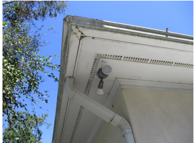
Typical gutter and downspout assembly
