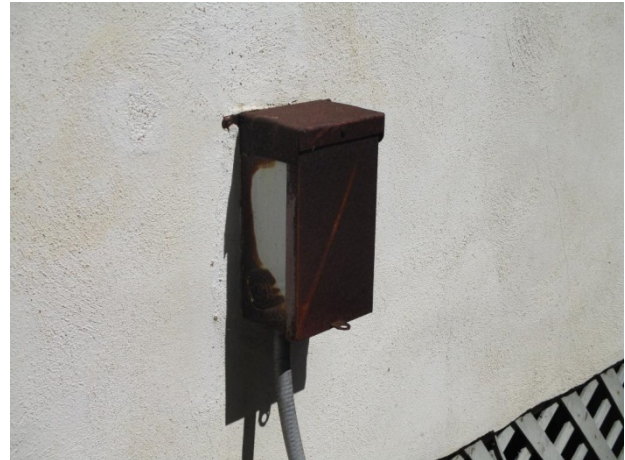
Rusted control box at condensing unit-maintain through operating budget
