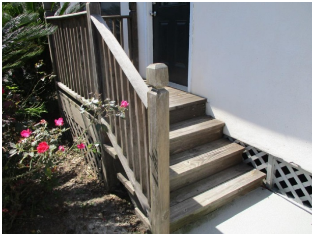
Deck at clubhouse entrance
