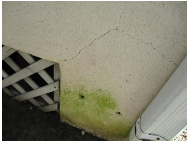
Stucco cracks and discoloration
