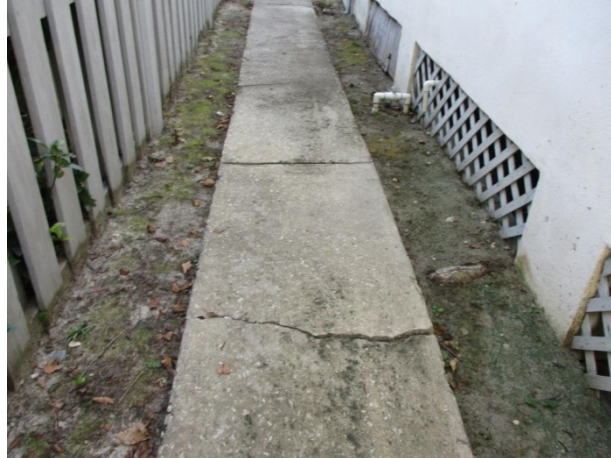
Sidewalk crack at the clubhouse
