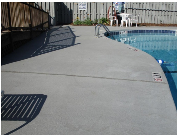
Pool deck overview
